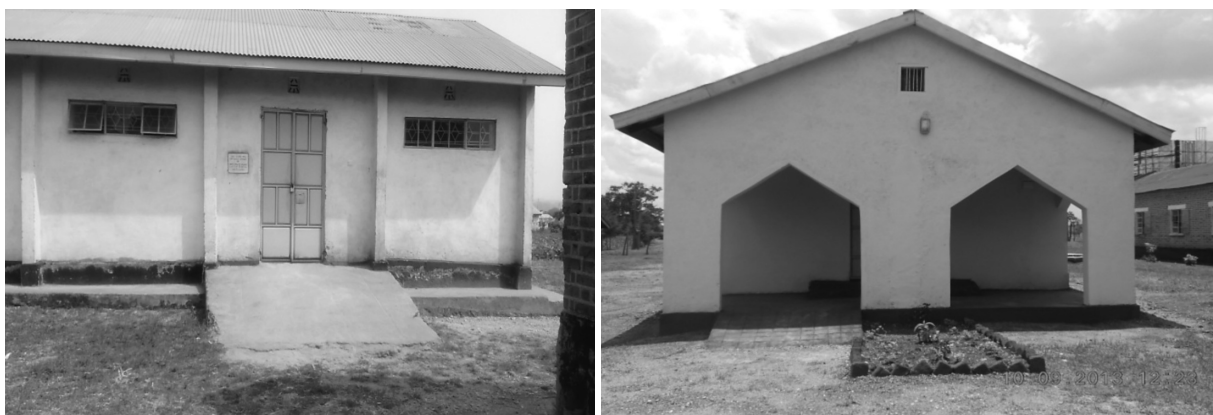
Prison buildings with ramps for accessibility by disabled offenders
